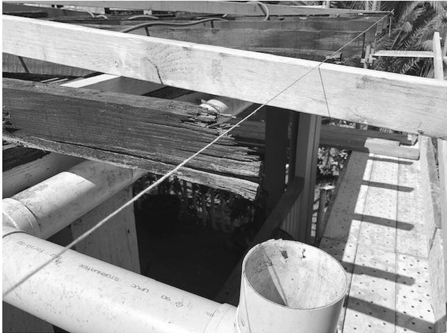
Rotten roof timbers once again. Entire front eaves also need replacing.
