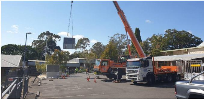
**Improvements around the parish—Air Conditioning at St Gerard's** is under construction, with the new gas powered condensers being lifted into place by crane this week. Repairs to the guttering and eaves at the back of St Gerard's will also be undertaken as part of the air conditioning installation
